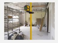
Using the STABILA LT 30 telescopic laser support, the LAX 300 G laser can easily be positioned at the desired working height.
