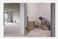
Avoid measuring and transferring errors when tiling with the STABILA LAX 300 G cross line plus plumb point laser – working directly on the laser beam. Quick and secure.
