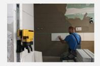
Tiling with the STABILA LAX 50 G cross line laser: work directly on the green laser beam – quickly and accurately.
