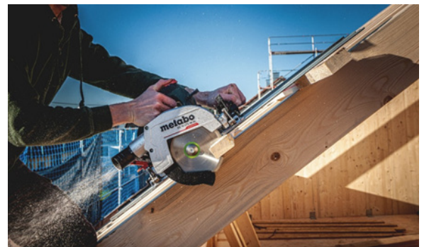
The new cordless circular saw KS 18 LTX 66 BL from Metabo achieves a cutting depth of up to 66 millimetres, and is ideal for mobile applications thanks to its compact and light design. Photo: Metabo
